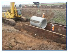
clay soil liner had eroded away over the last 60 years, and as much as 43 percent of the water was seeping out. The flow was also being slowed by bank erosion, debris and dead timber. Combined, these factors reduced the efficiency to less than 45 percent of original design capacity.
